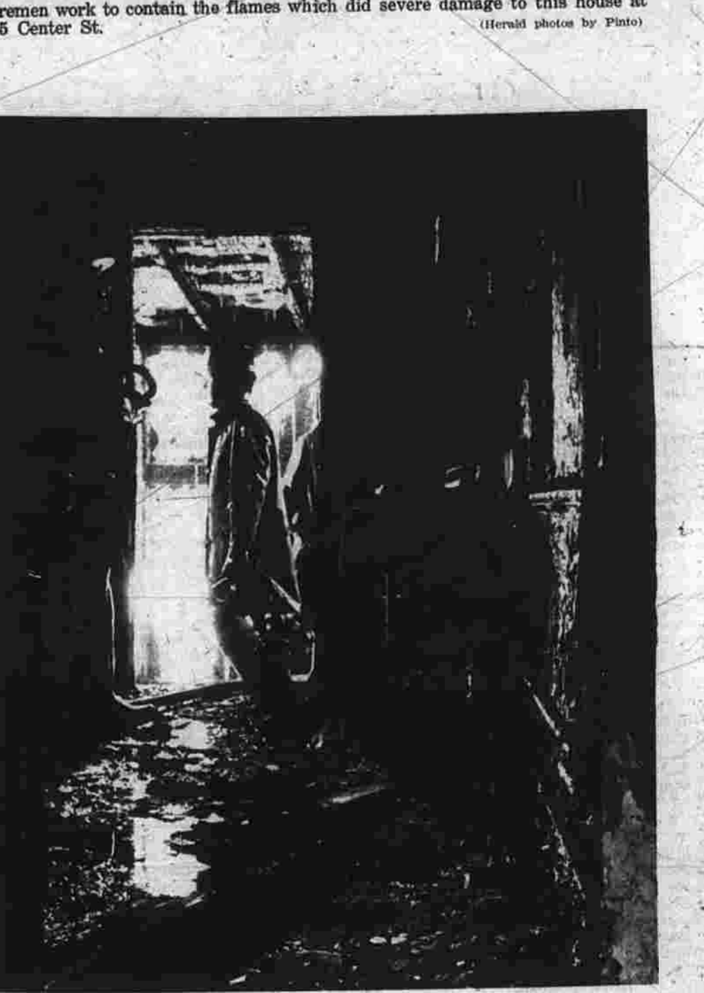
The rear of the second floor, just inside the porch, was gutted.
